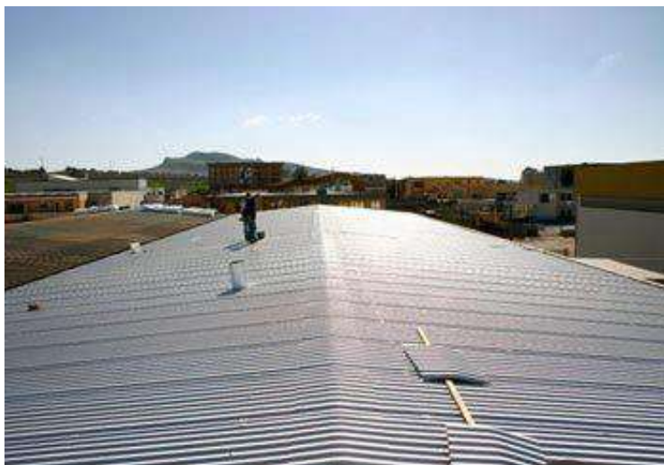
Figura 32: POST-OPERAM (COPERTURA IN PANNELLI SANDWICH)
